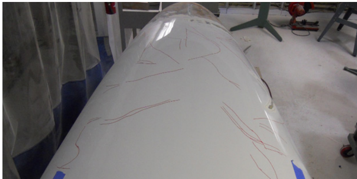
Visible paint cracking on a composite surface.
